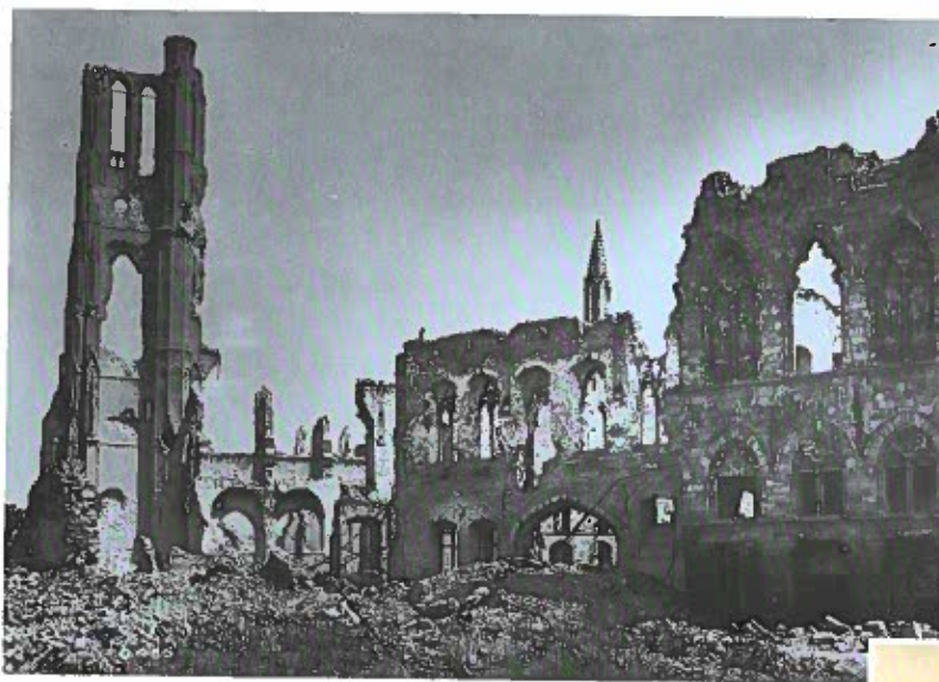
The Tower, St. Martin's Cathedral, Ypres, Belgium, damaged by the war. RIGHT: A Canadian soldier tends to a tiny victim of the war.
